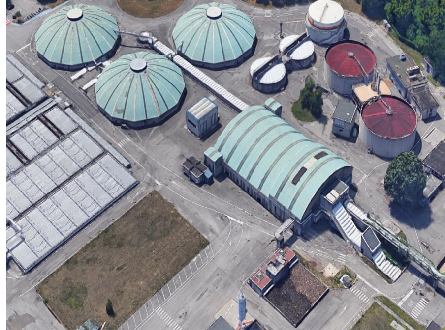
3 large primary covered circular sedimentation tanks
