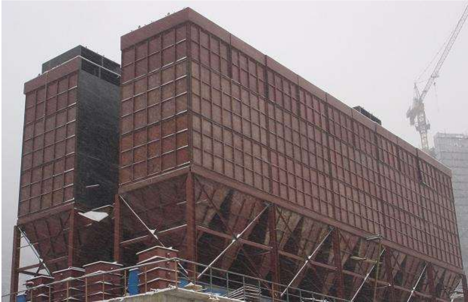
A 20-compartment baghouse at a cement processing plant.
