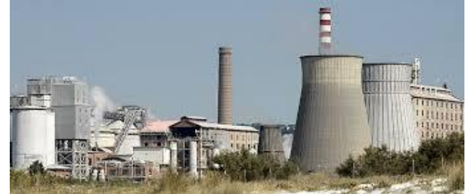
Solvay plant at Rosignano (Tuscany, IT)
