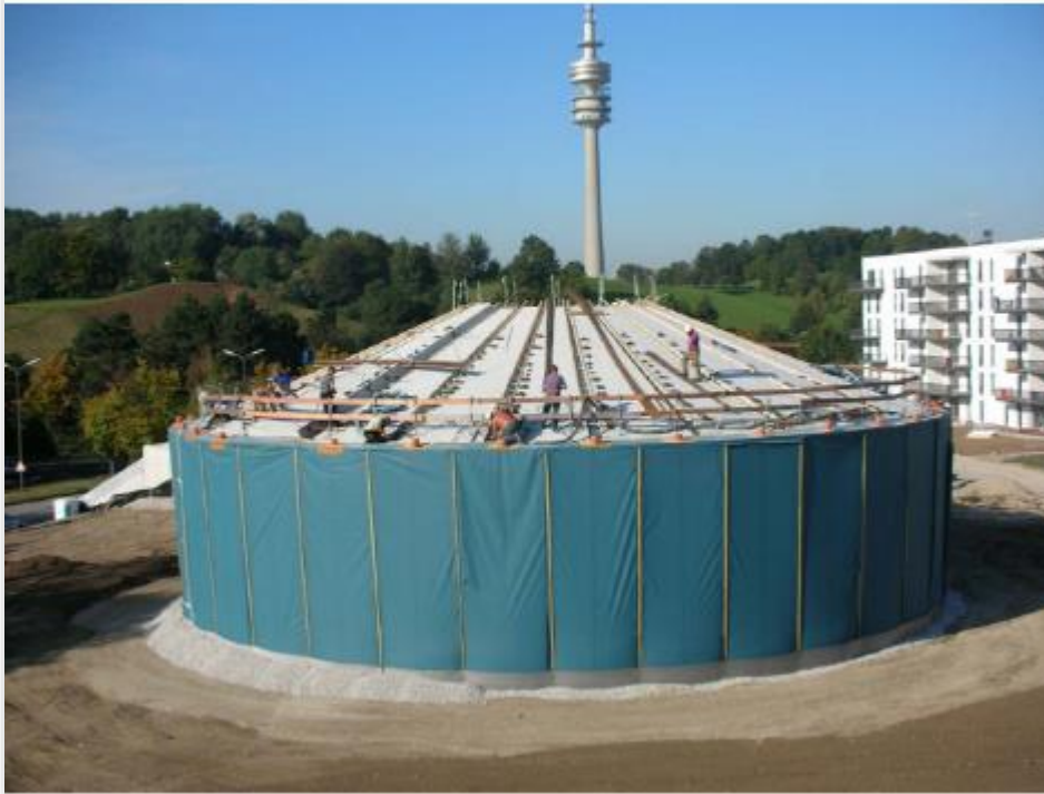
Munich: Realization of tank thermal energy storage
