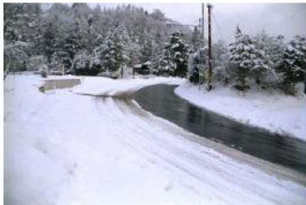
Fig. 3 Snow-melting condition at the upper section of the road on Feb. 13, 1996.
