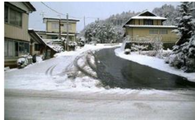
Fig. 4 Snow-melting condition at the lower section of the road on Feb. 13, 1996.
