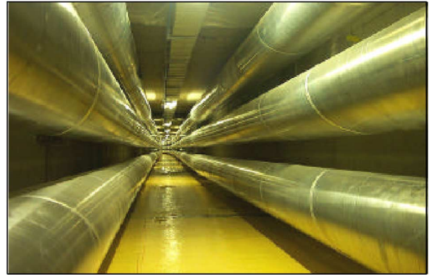
Fig. 2. A 300-kV double-circuit GIL in PALEXPO (Switzerland) Geneva Airport tunnel (in service since 2000, Siemens).
