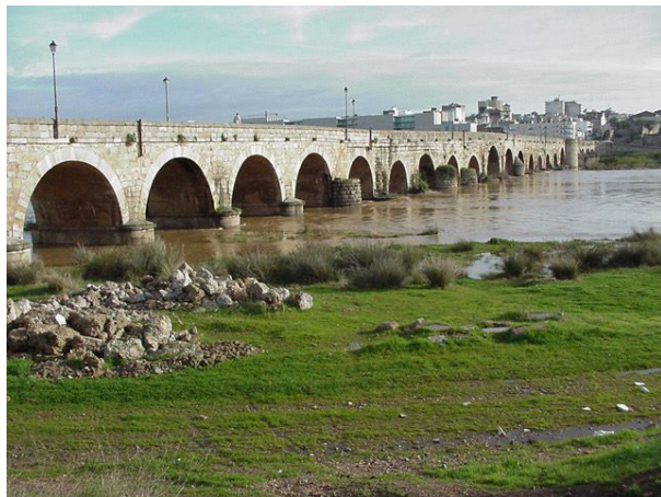
Roman Bridge. Barrel vaulting, River Guadiana.
