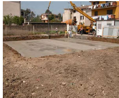
It is a concrete poor in cement with poor mechanical characteristics used as backfill of the sub-foundation
