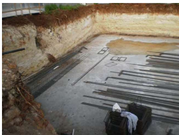
It is a concrete poor in cement with poor mechanical characteristics used as backfill of the sub-foundation
