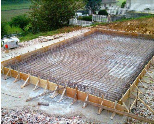
Before concrete pouring
