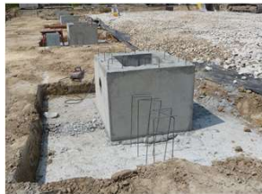
On site construction
